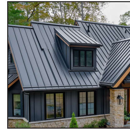
STANDING SEAM METAL ROOF COLOR: SLATE GRAY
